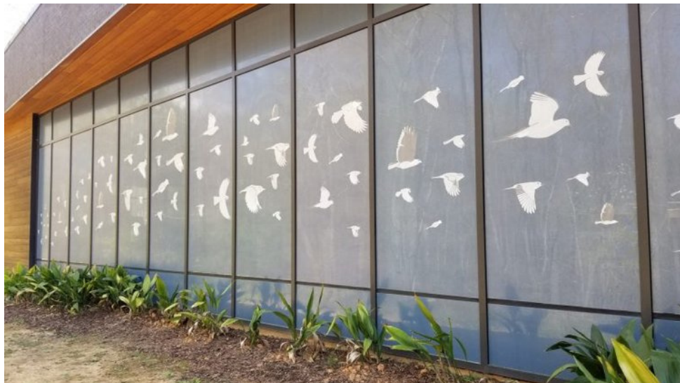
CollidEscape window film installed at Richland Library Ballentine prevents bird strikes, and it is transparent from indoors! Image courtesy of Richland Library.
